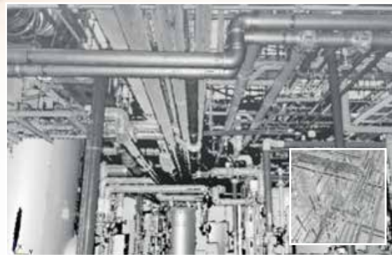
Point cloud data on pipes in a plant
