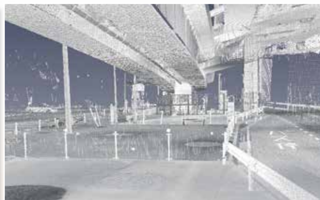
under a girder bridge
