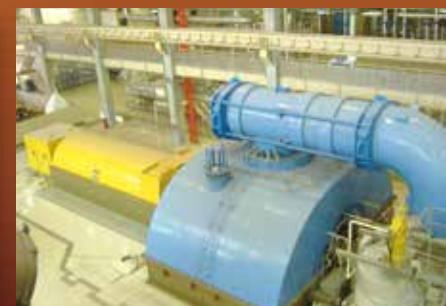
Power generation facilities
